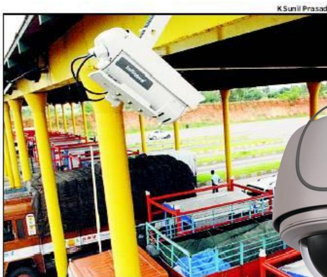
Created for NICE (Nandi Infrastructure Corridor Enterprises), Infinova IR illuminated day/night IP65 cameras monitor lanes, IP PTZ cameras and fixed domes monitor traffic at plazas
